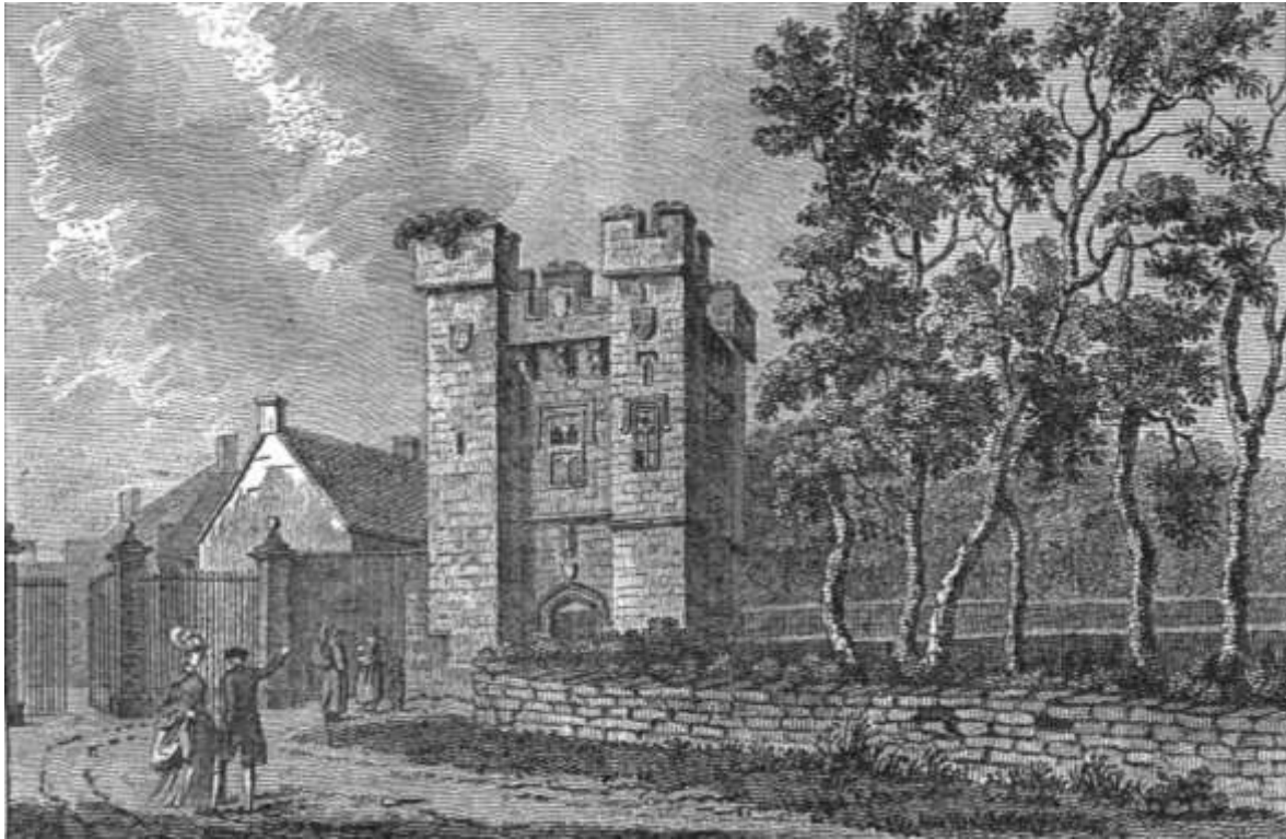
Figure 2: Alnwick Abbey, view showing the Gatehouse c. 1773
